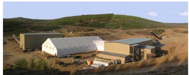
The Minto mine – ore storage and mill structures
